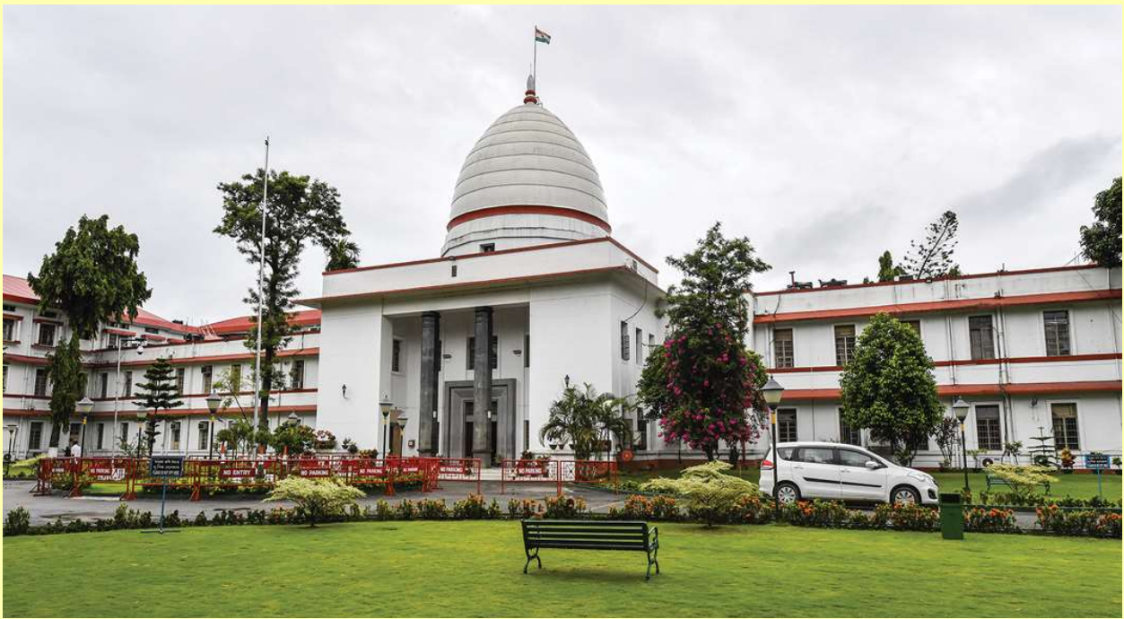
The Gauhati High Court building (now old block) opened by Shri Govind Ballabh Pant, Union Home Minister, on 20 th February, 1957
